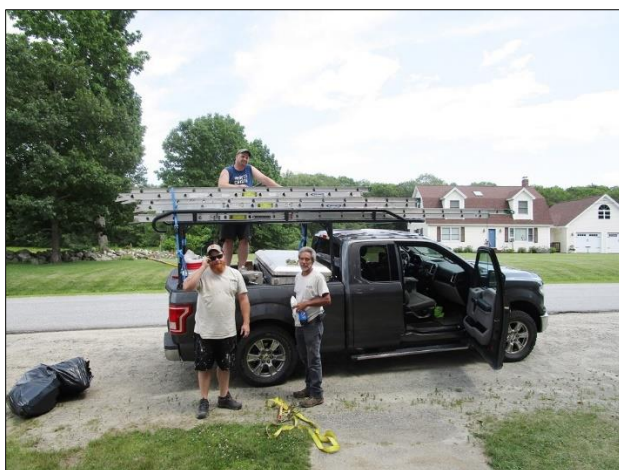
The steeple repair is completed! Above: Mid-Maine Restoration packing up on their final day. The church bell was rung in celebration!
