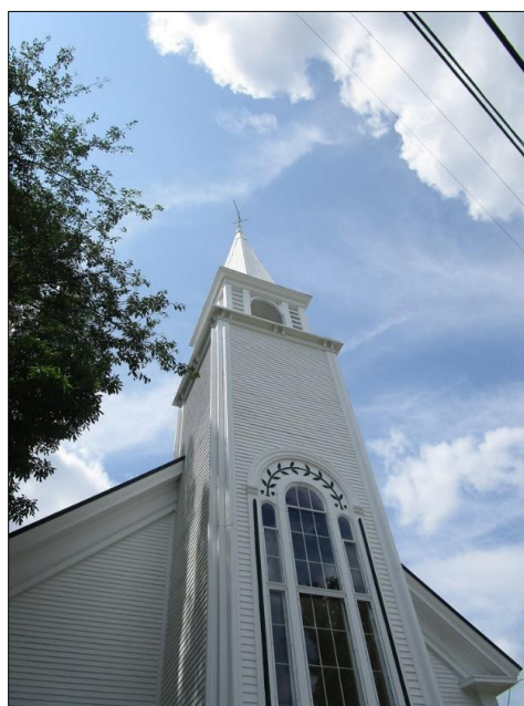
The newly restored Edgecomb Community Church steeple!
